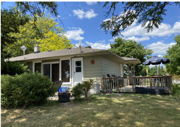
PHOTO 5: View of the southern portion of Building D facing north located on the east advanced property.
