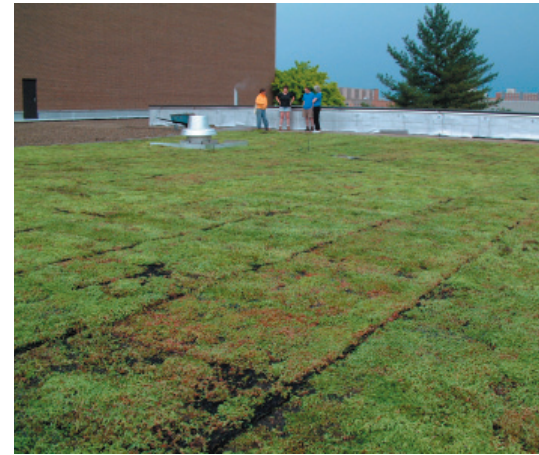
Photo 29: This flat roof is planted with grass which reduces local temperature and retains water.
