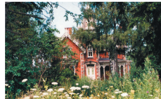
Photo 12: Character properties reflect Milton's cultural heritage and should where feasible be integrated into the developing community.
