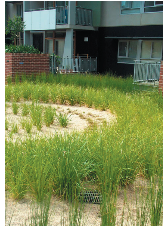
Photo 25: This swale filters rainwater, prevents run-off and ensures slow percolation into the ground.
