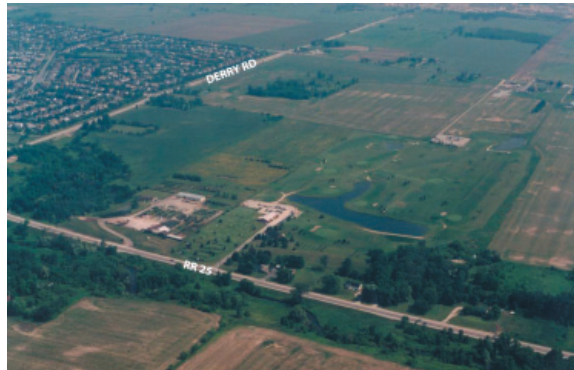
Photo 5: View south west at Regional Road 25 East
