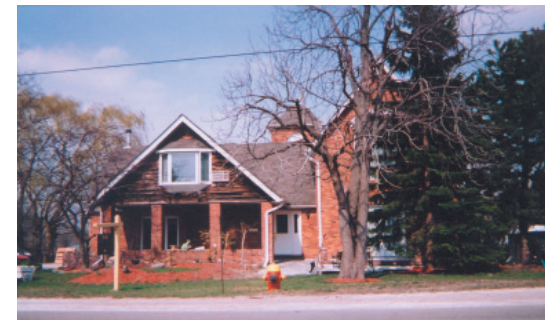
Photo 15: Existing brick farmhouse on Main Street
