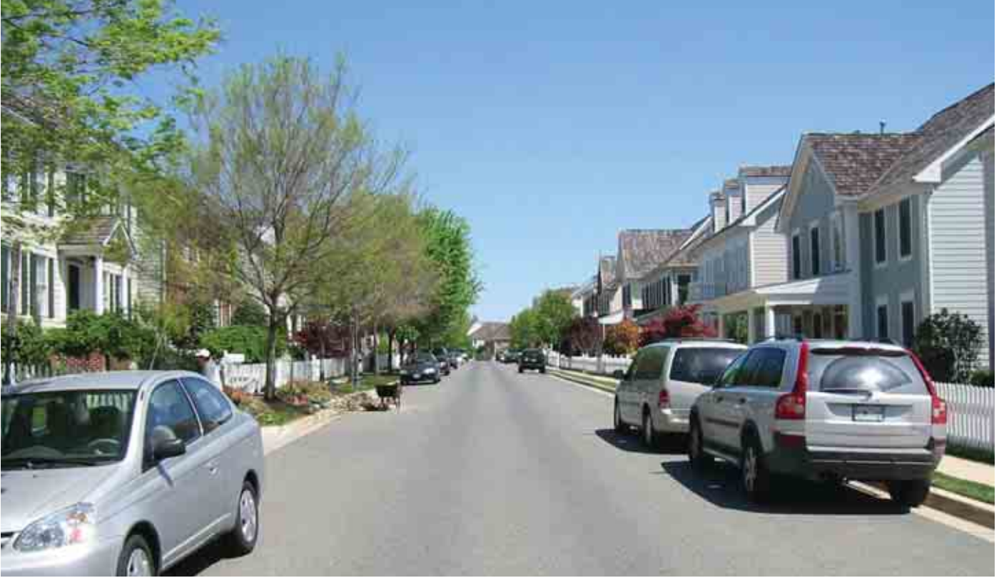
Local Roads should be designed as pedestrian scaled streets. On-street parking narrows the street width, reduces vehicles speeds and provides a buffer between pedestrian and vehicle traffic.
