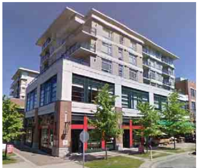
Taller buildings should step back above the building base to reduce the perceived mass of the building.
