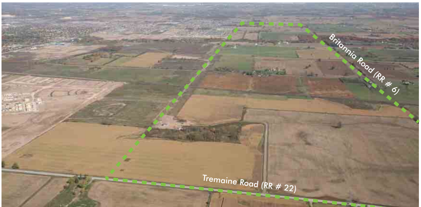
An aerial view of the Secondary Plan Area, looking northeast from Tremaine Road.
